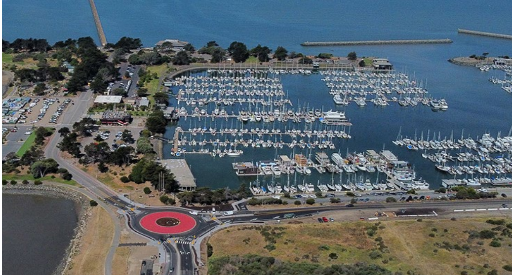
Figure 5: Concrete slab inside Marina just above red traffic dot serviced old ferry, and is innermost location. D&E dock location is much closer to entrance, out of sight in image but on far right about halfway up. K dock extends from the harbormaster's office in center of marina. The Hornblowers dock by the hotel on far right (not shown) in the marina. Source: https://berkeleyca.gov/your-government/our-work/capital-projects/waterfront-specific-plan
