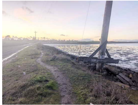
Above: Gouges and erosion along Virginia Extension
