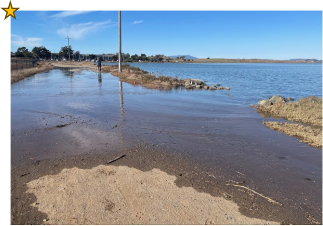
Existing Flooding Occurring at King Tide
