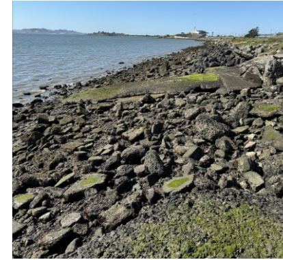
Concrete Debris Shore
