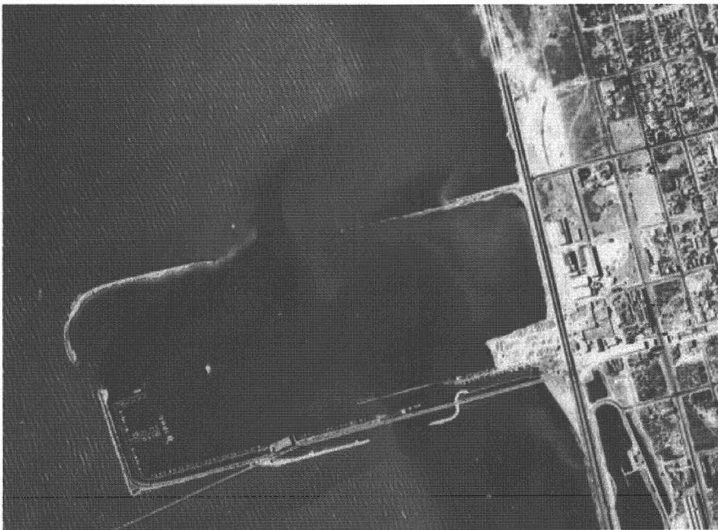
1939 Aerial view of recently completed Berkeley Yacht Harbor. Former Golden Gate Ferry pier is narrow structure that extends out of picture at lower left and the Berkeley Municipal Wharf is at the east end of that pier, offset, on the south side of the new harbor jetties. (Photograph: UC Berkeley).
